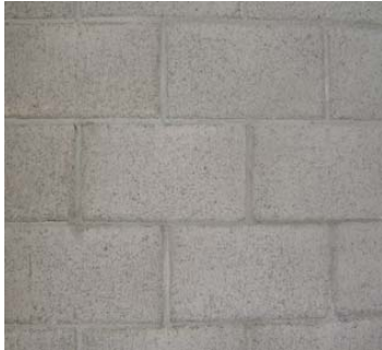
Surface 1 – Bare Wall
