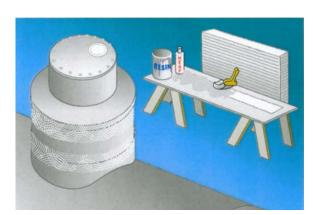
Wet-out or soak, with brush, liquid resin over fiberglass mat. Mat will go clear when fully saturated. If additional resin is required, use only resin from Western Fiberglass, Inc. The resin used in construction of all Western Fiberglass, Inc. components is corrosion resistant resin, made for use in fuel and chemical applications.
